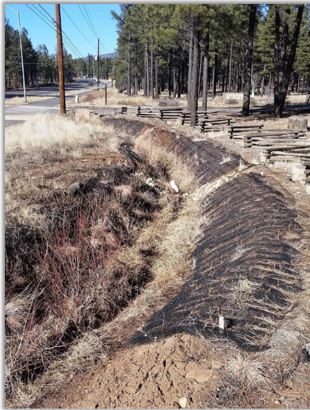
Figure 4: Turf Reinforcement Netting at Downstream End Looking Northwest
